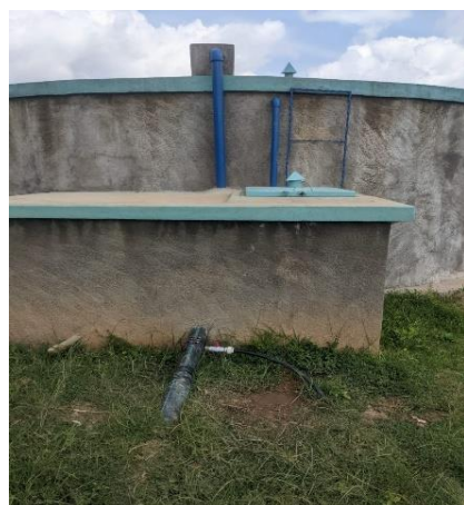
Figure 3: Water tank rehabilitated /Tare Sector/ Nyamagabe District
