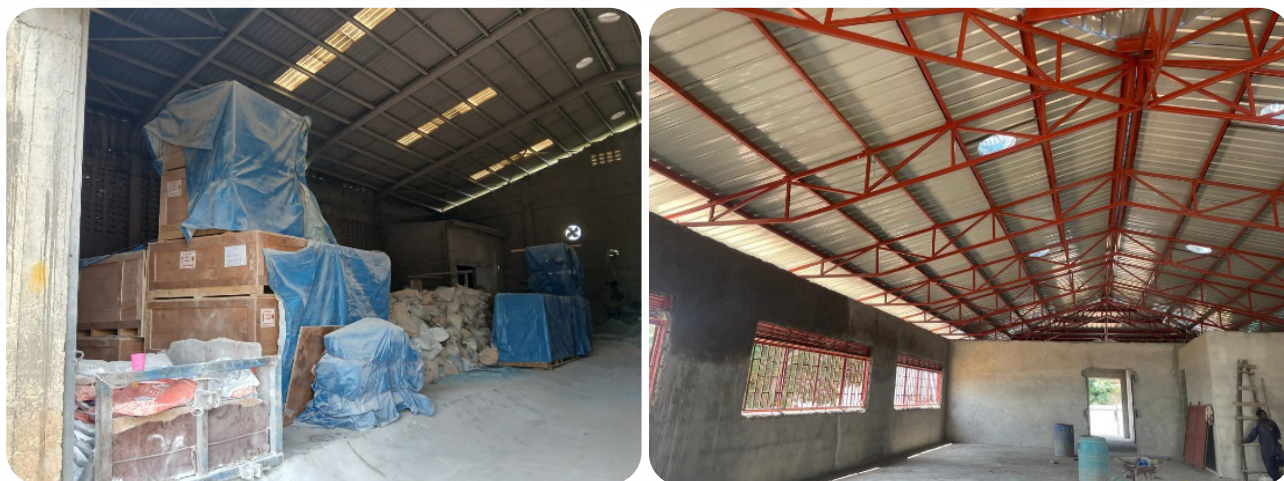
Figure 10: Equipment in storage at contractor's warehouse and Construction of calibration house in final stages at Entebbe
