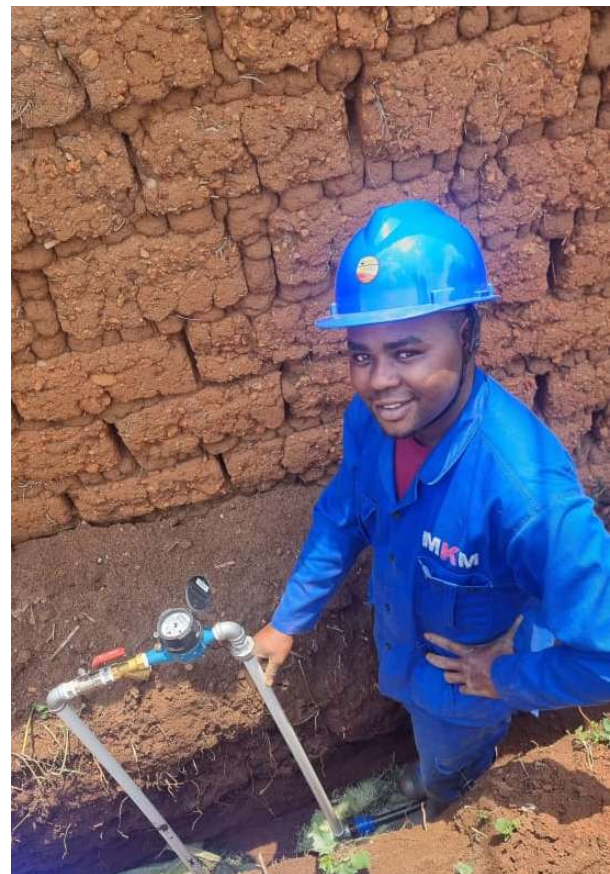
Figure 12. MKM team member poses with a newly installed household water meter
