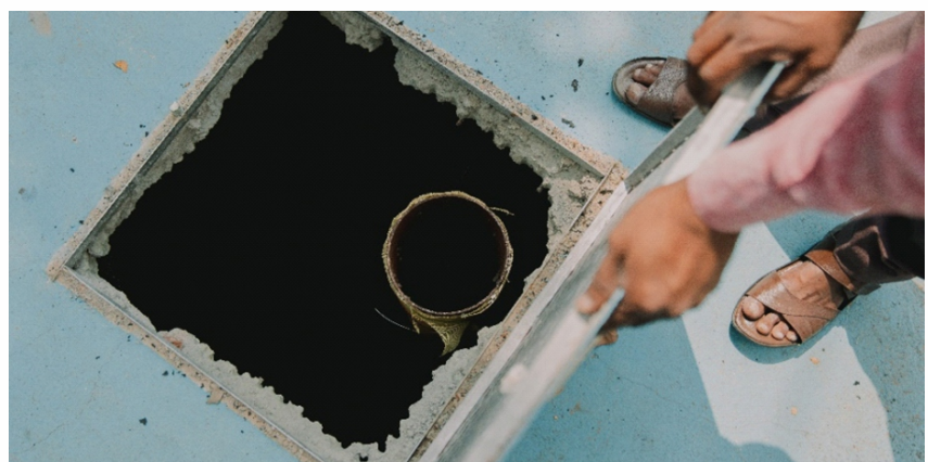
Abandoned borewell converted into recharge structure
