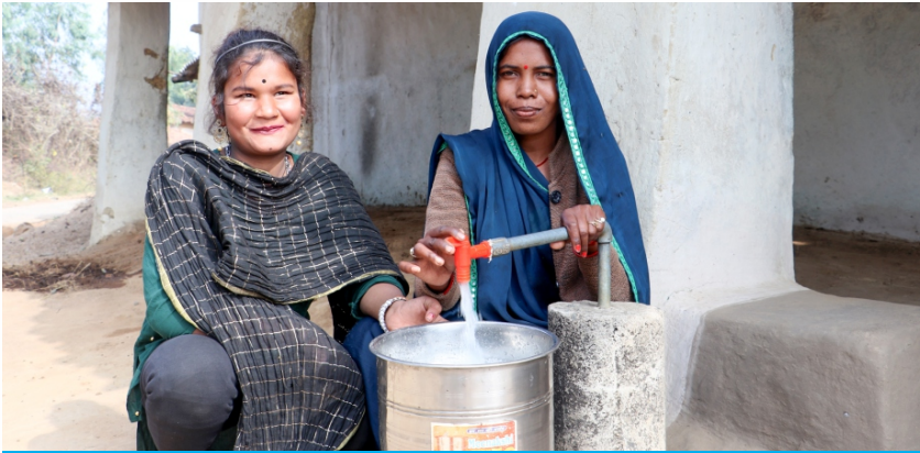
Rajkumari Singh of Sontola village, Harrhatola Gram Panchayat taking water from the household tap installed in front of her home under GMVRSS, dated 10 th February 2024
