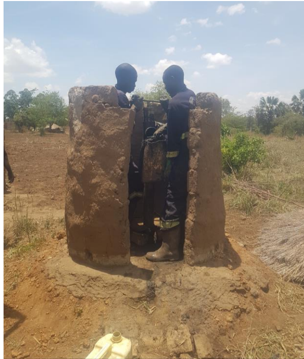
Figure 9: Pit Emptiers Emptying Latrine using the Gulper IV
