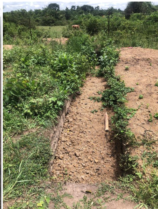
Figure 17: Backfilled Trench
