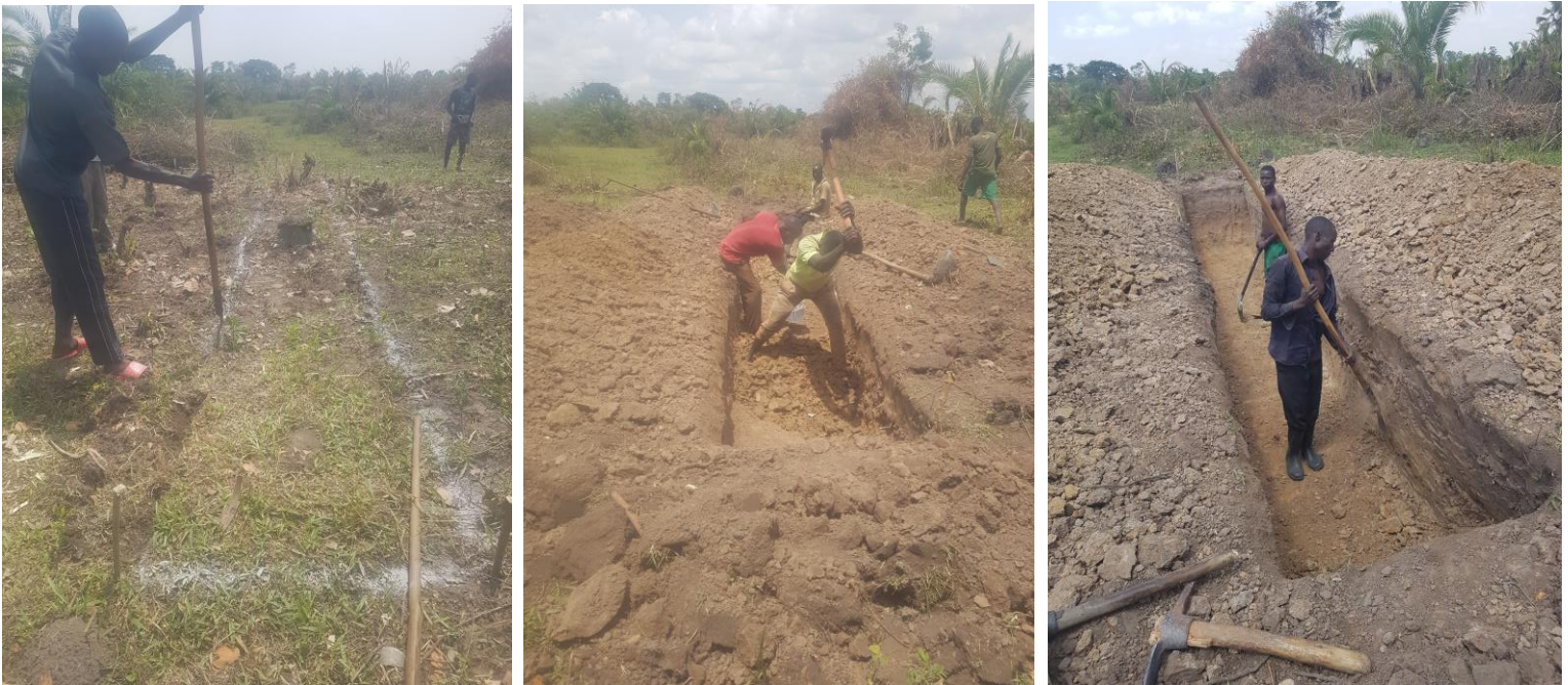
Figure 13, 14 & 15: Trench Layout and Excavation
