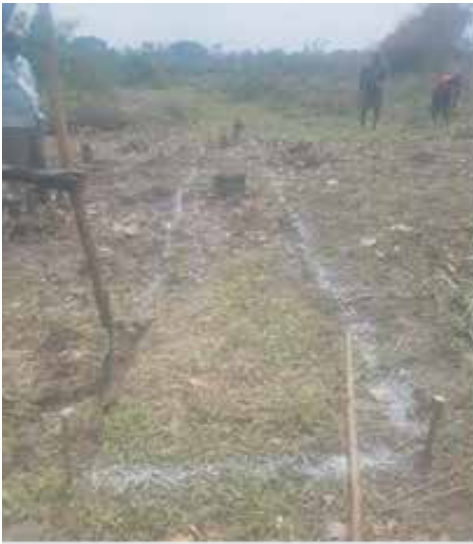
Picture 5,6: Trench Layout and Excavation
