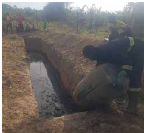
Picture 8 & 9: Pit Emptiers emptying FS for the first time in the trenches
