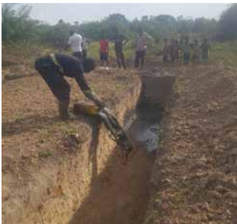
Picture 8 & 9: Pit Emptiers emptying FS for the first time in the trenches
