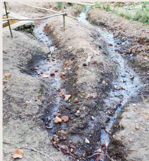
PHOTO 6: Trenches diverting dirty running water away from water source
