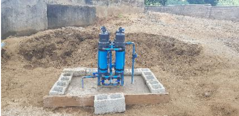
A chlorine dosing unit at Limphangwi during construction
