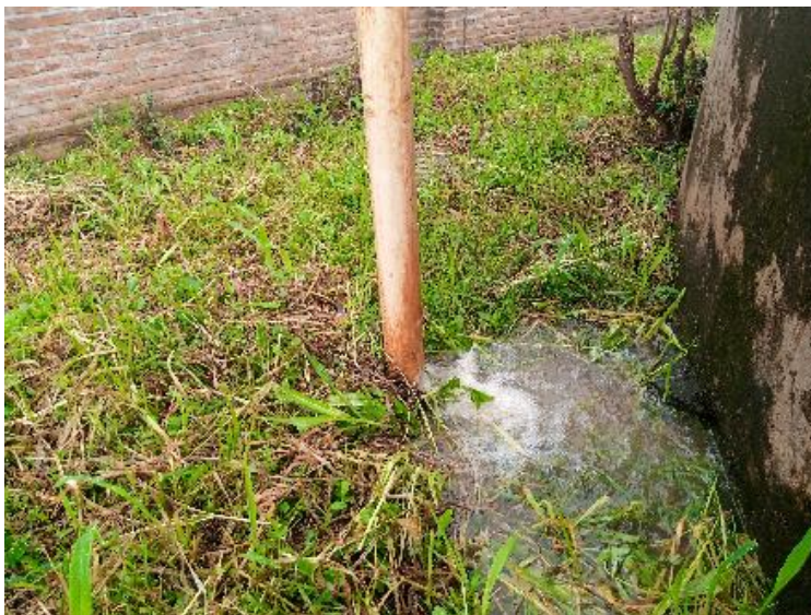
An unattended fault at Mbadzi
