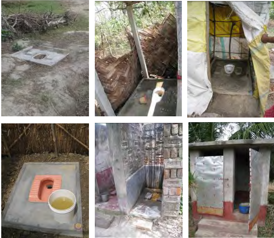
Photo 2: Differing quality of top-structures: from none, via reeds and plastic to bricks and concrete
