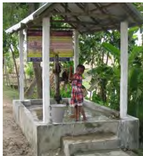
Photo 4: Typical design of a water point with raised platform and a protecting roof, in Mahendragunge
