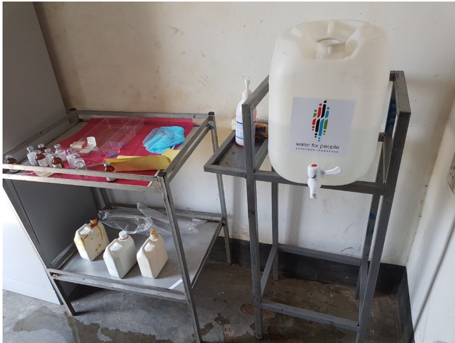
Photo 2: A handwashing station installed in one of the treatment rooms at Bwiizi Health Centre III by Water For People
