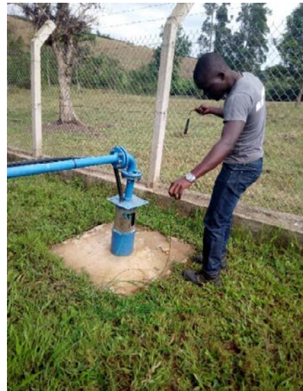
Figure 4: installation of the diver into the well after downloading
