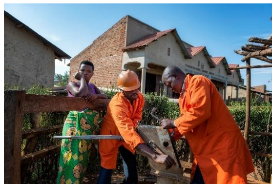
Photo 7: Hand Pump Mechanics repairing one of the boreholes on the pay-as-you-fetch model in Kabambiro as the caretaker looks on
