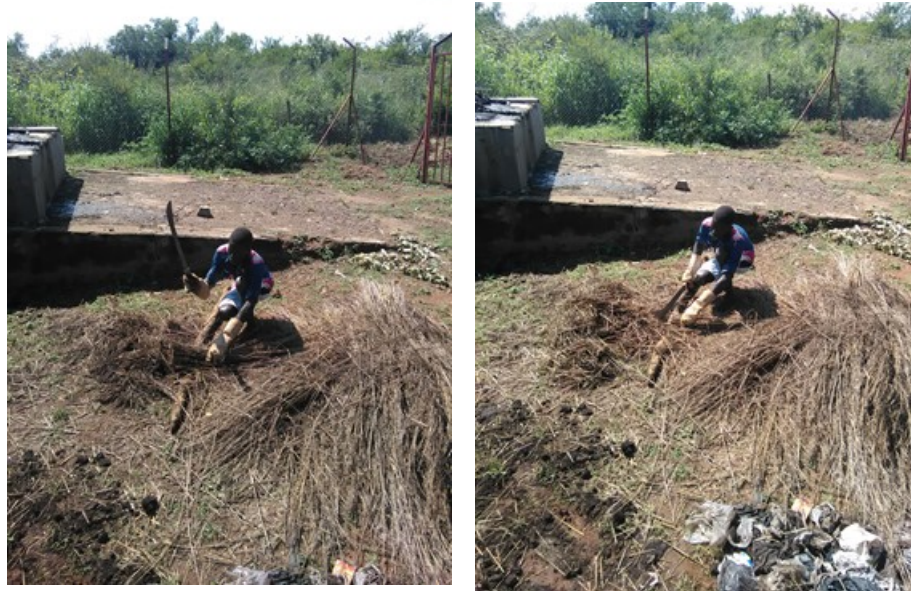
Figure 4: Preparing the structure support material
