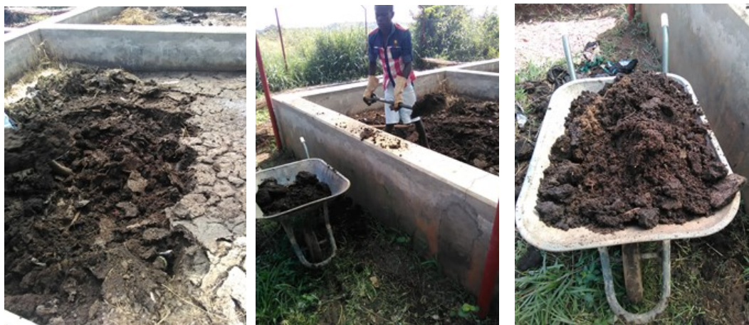
Figure 3: Removing sludge from drying beds
