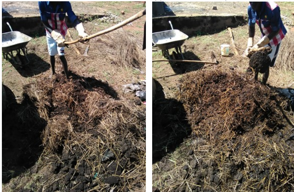
Figure 5: Mixing sludge with structure support material
