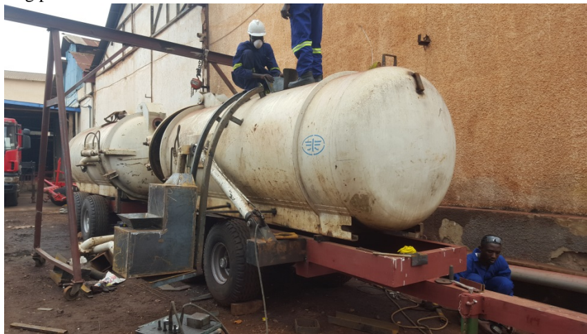
Photograph 1. modification of vacuum tanker to a transfer tank
